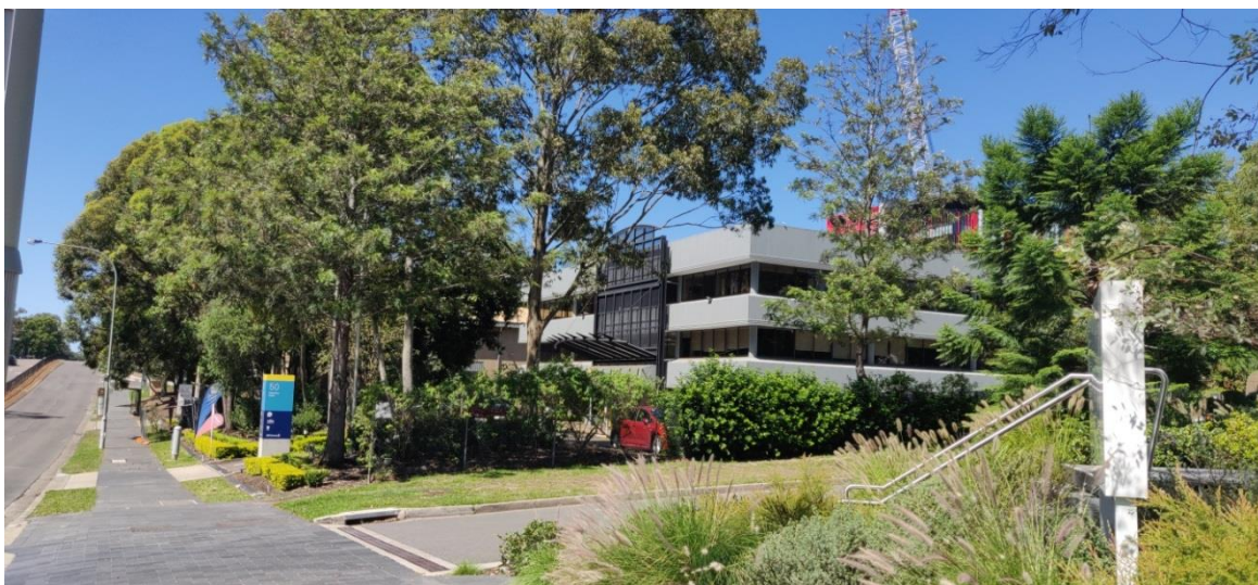
Figure 6. Existing commercial office building at No. 48 Waterloo Road.
