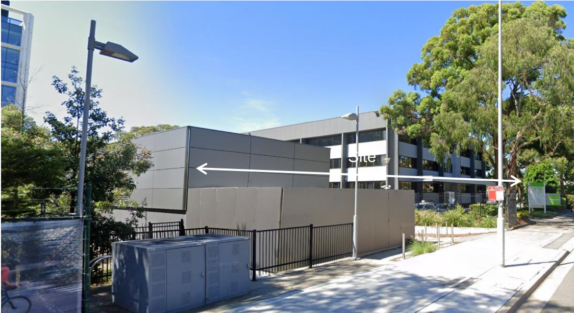
Figure 3. Macquarie Park Station fire egress stairs, ventilation shaft and bike storage, and a 3 storey commercial office building to the south-east of the site.
